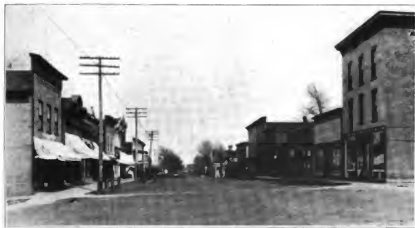
CITY WATER WORKS, CLARENCE EAST LOMBARD STREET, CLARENCE
